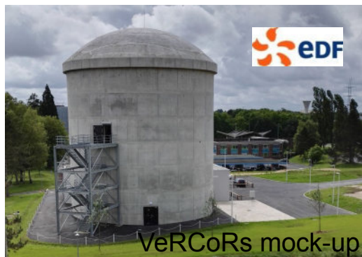
Legland J.-B. et al, Evaluation of crack status in a meter-size concrete structure using the ultrasonic nonlinear coda wave interferometry. JASA , 2017
