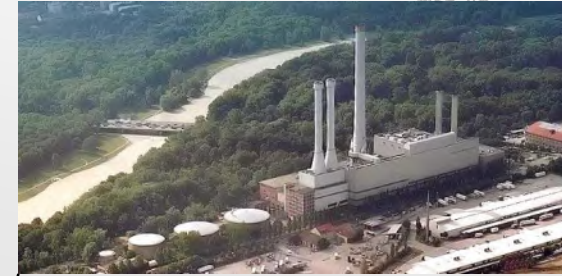
Geothermal power plant
